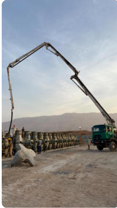
Figure 6: Concrete pump transferring fresh concrete into the CORE-LOC™ mould.
