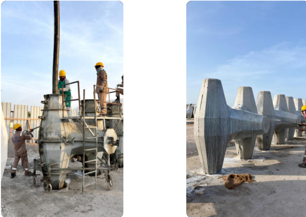
Figure 7: Concrete casting into the CORE-LOC™ mould, and curing compound application after demoulding.
