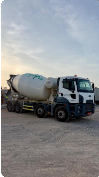
Figure 5: Ready-mix transit truck delivering fresh concrete to the casting yard.
